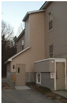
New elevator dedicated 1999 thanks to the many donations of Church and Community.
